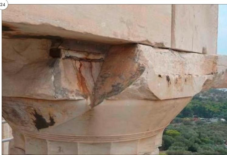
Corrosion of an iron connector led to cracks and outburst, Acropolis, Athens
