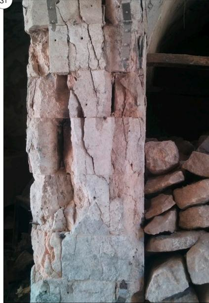
Excessive heat can seriously damage the stone structure, causing cracks, chipping or outburst Suq as-Sabun, Aleppo
