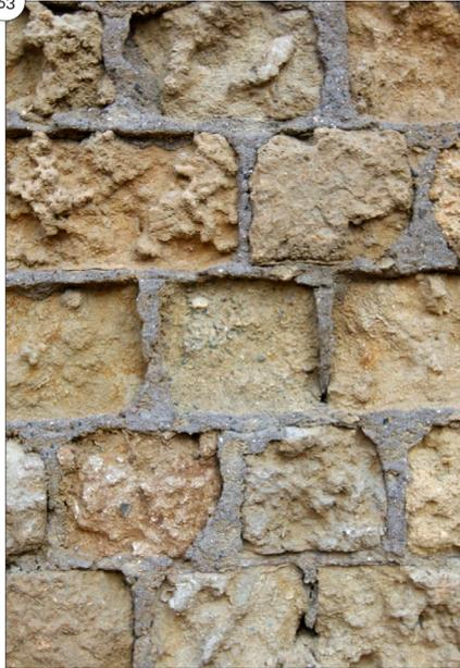
Sandstone with cement mortar joints, leading to detachments, Cordoba, Spain
